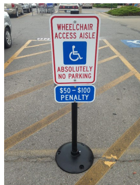
For Quantitative Study One, the researchers added signs and “No Parking” pavement markings to the access aisles at one site. This access aisle warning sign is patterned on South Dakota’s.
